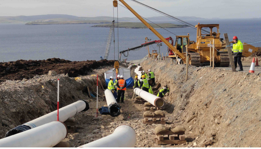
Oil pipelines being laid in Shetland, photo: shetnews.org (left) and a pig (Pipeline Inspection Gadget), photo: Wikimedia Commons (right)
