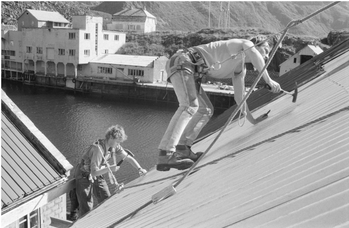
Photo taken by Wolfgang Eschenhorn, Roofing Work, 1987.
